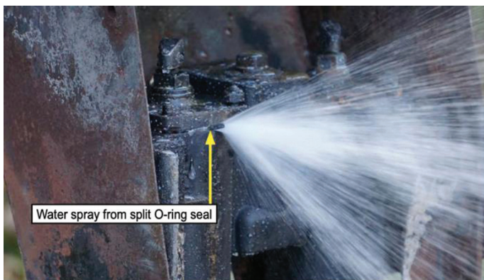
Post-accident test using water to simulate fuel spray
