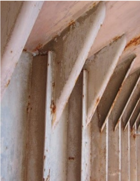
Cargo residues remaining on the framework
