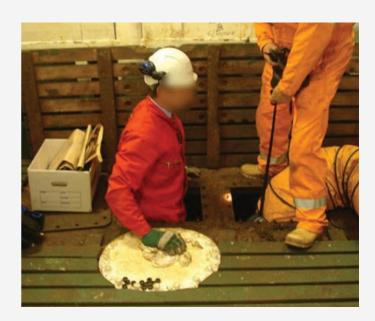
The restricted manhole opening into this chain locker made it difficult to access the space whilst wearing SCBA and to recover the persons who had collapsed inside
